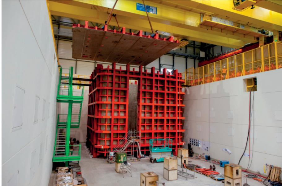
Figure 1.10 – Assembly works carried on the external frame that will host the liquid-argon chamber of NP-04.
