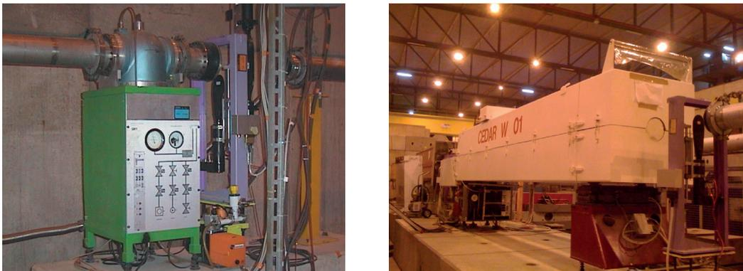
Figure 1.18 – Left image: CET monitor with gas pressure control system. Right image: CEDAR installed in a North Area beam.
